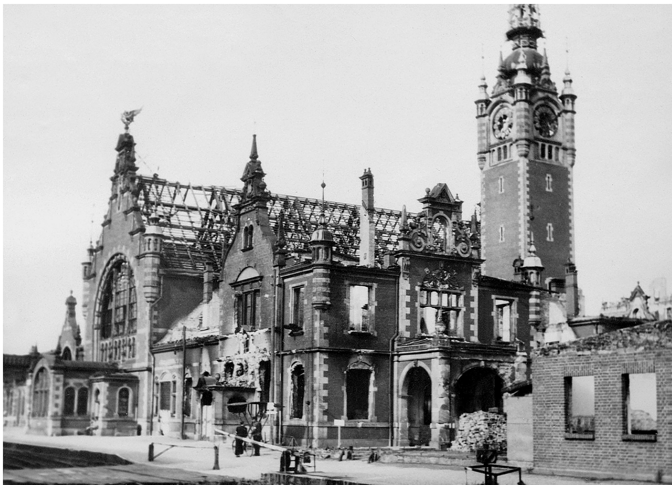
The Main Station in Gdańsk, destroyed during the war
